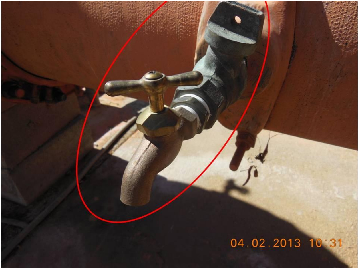
Figure 1, installation of a smooth-noosed sample tap/bib at well 1 (W01; correction to SDWIS ID 12; photo by Wild Earp, Acme Water System).
